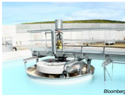
Main picture: A binding agent mixed with sea water, attracts the foreign matter in the water in the first stage of the desalination process at the Thiess Degrémont, Victorian Desalination project in Wonthaggi, south east of Melbourne, Australia.
