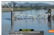
Fixing America's Falling Infrastructure Q
